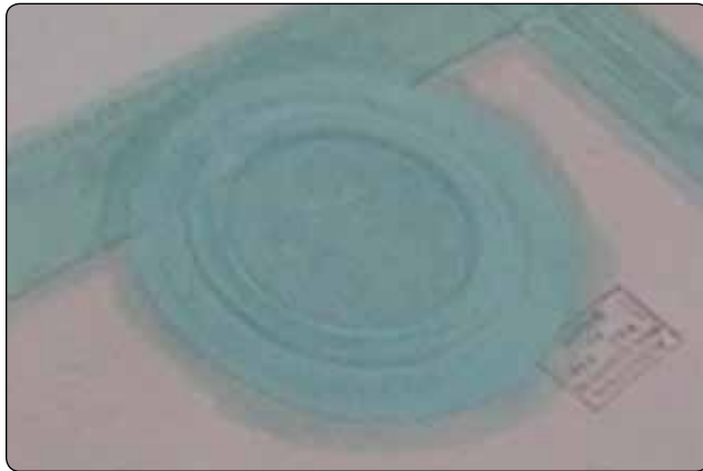
Figure 3-30. This inspection ring was cemented into place on the fabric covering. The approved technique specifies the use of a fabric overlay that is cemented over the ring and to the fabric.
